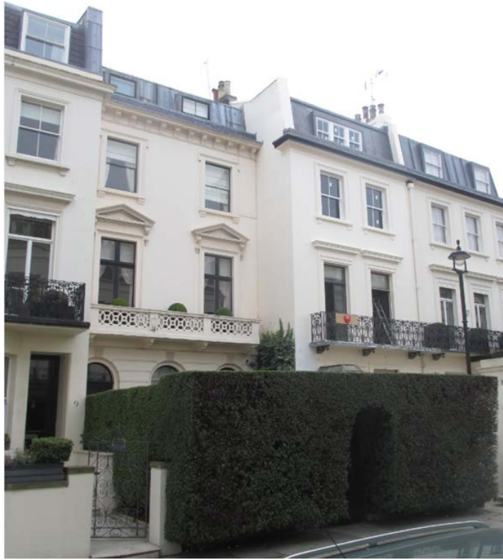
To the front 11 Gerald Road
